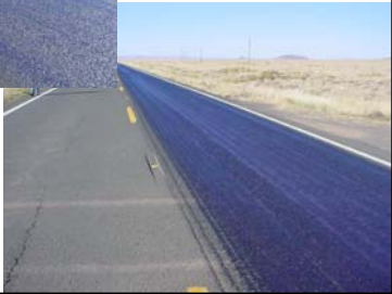
SR 264 Flush coat - seals up the pavement and extend its life
