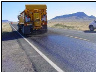
SR 264 Flush coat - seals up the pavement and extend its life
